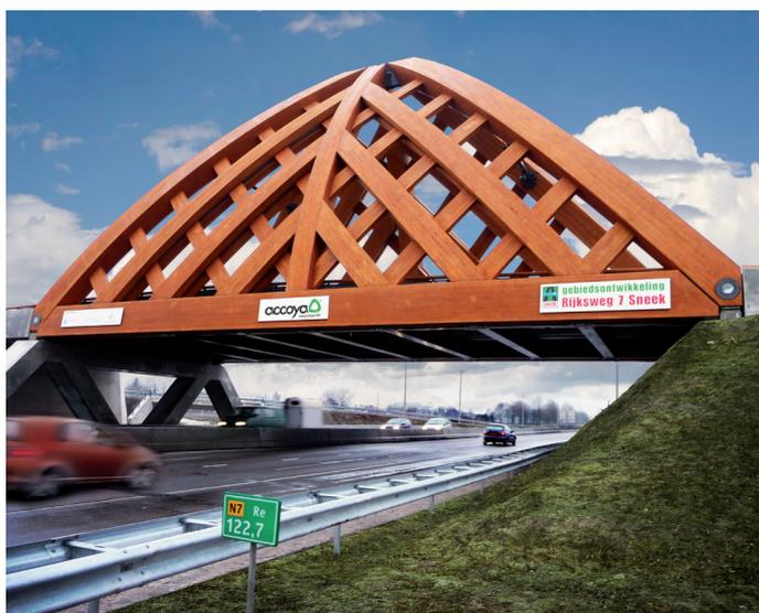
**Figure 7:** A large scale application of Accoya® wood – Sneek bridge, the Netherlands
